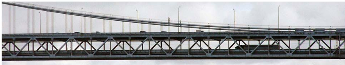
Detail of Oakland Bay Bridge, San Francisco, USA 2008.
