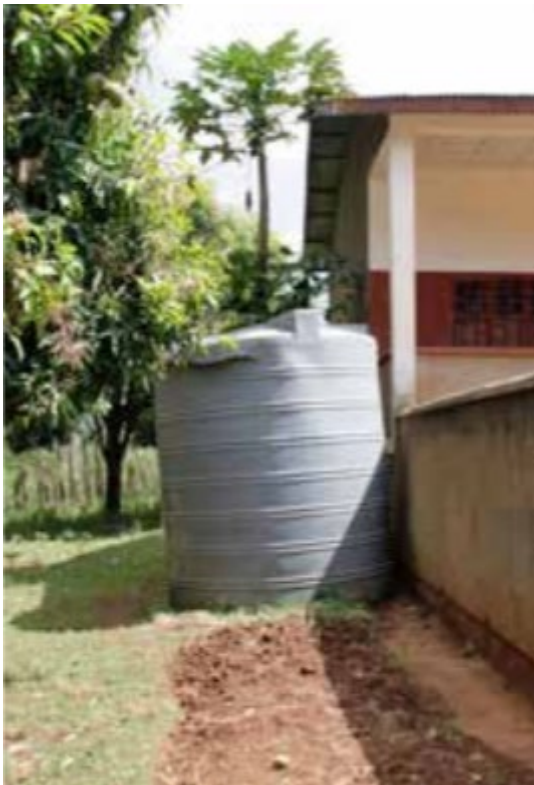
In the future, the spring water will be available at the school in this 10,000 liter barrel (Bildunterschrift)
