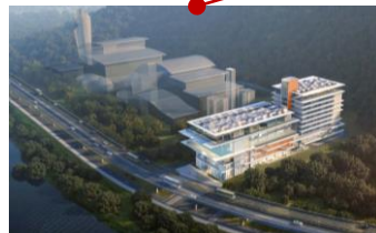
Sport Center, Nanshan District, Shenzhen 深圳南山垃圾发电厂的文体中心
