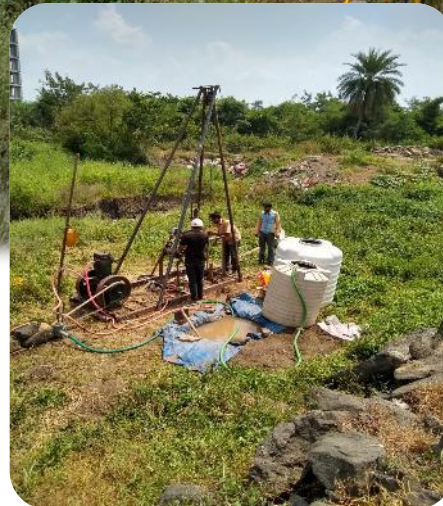
Bore Hole @ Culvert Locations
