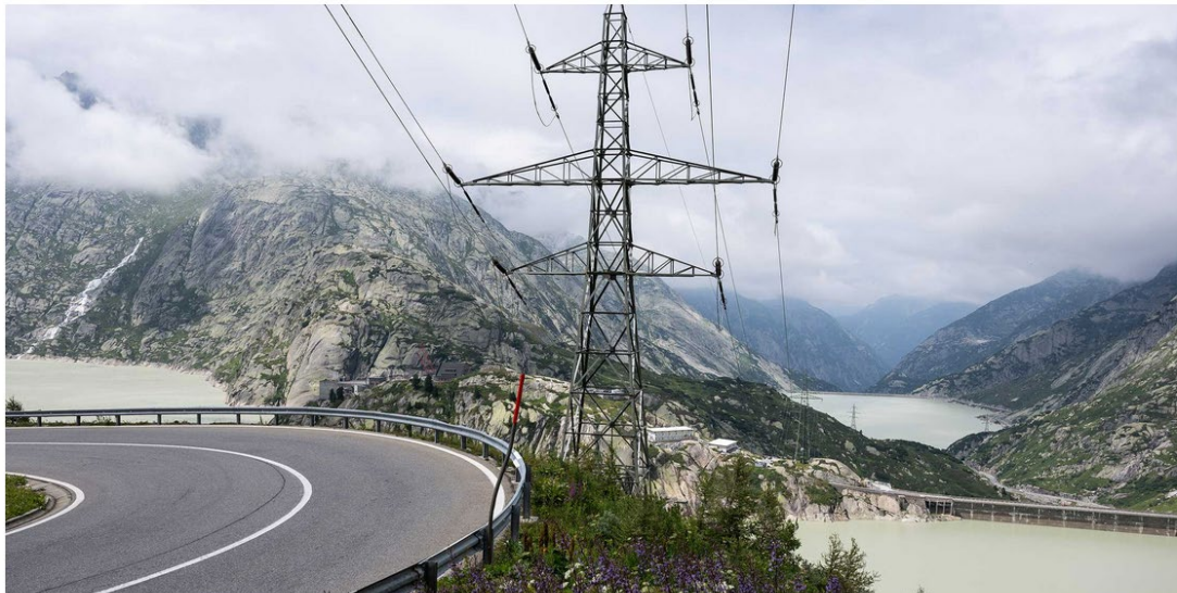
Swiss reservoirs such as Lake Grimsel make a significant contribution to the resilience of the Swiss electricity system to shocks. (Photograph: Peter Schneider / Keystone)
